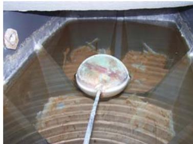
Slime (or biofilm) can occur in tanks and pipework and this can provide a safe haven for legionella to grow. It is therefore important to check tanks for slime as well as obvious dirt and debris on the tank floor.
